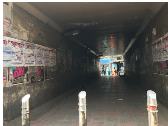
NEED FOR INTERMEDIATE NATURAL OR DAYLIGHTING IN PEDESTRIAN UNDERPASS
